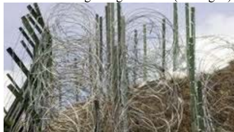
Fig.1 Photograph of fence along LOC
