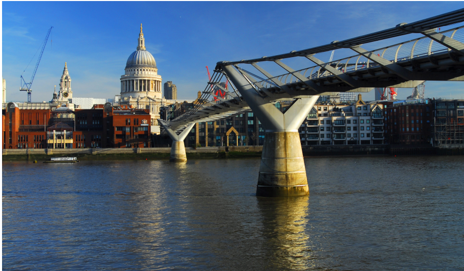
Figure 19: The London Millennium Footbridge [LRP07].
